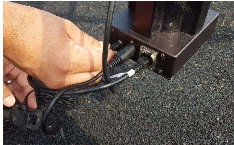
26. Attach Cat6 cable from extender behind monitor, pan tilt remote, and LANC remote that controls the camcorder zoom and record functions, to the base of the tower.
